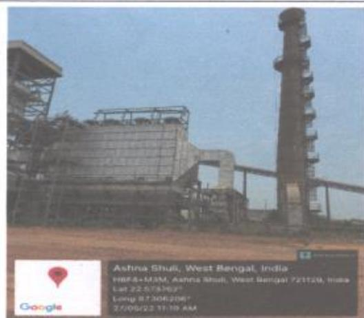
**ESP ATTACHED TO CPP (Photograph-3)**
